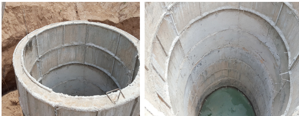
Figure 8 Lining of the collapsing loose walls (such as in sandy soils) using ring walls in the construction of HDWs
