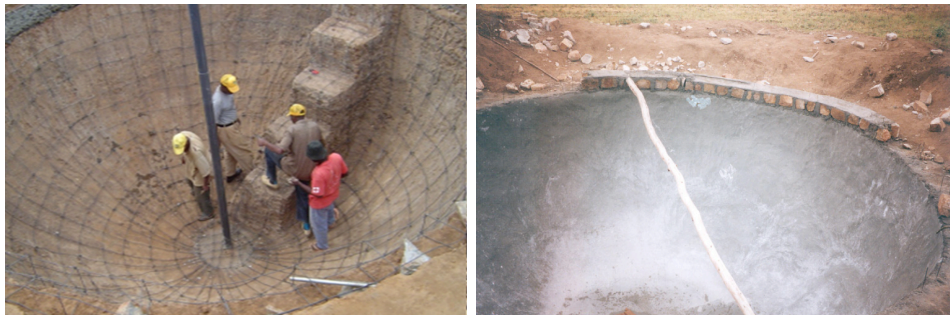
Figure 3: reinforced concrete lined pond under construction
