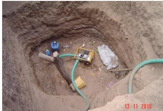
Figure 20 manually drilled tube well installed with diesel engine pump
