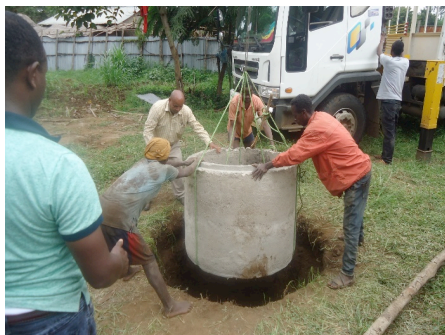
Figure 13 Perforated concrete casing
