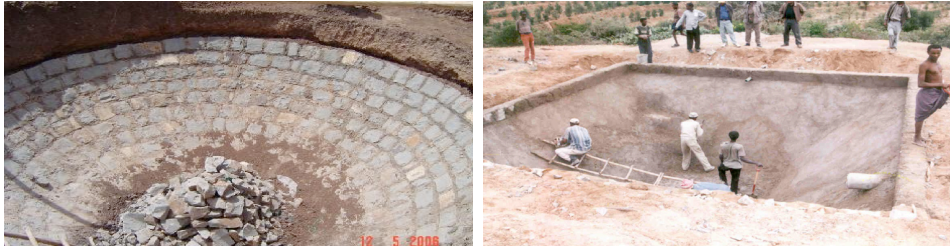
Figure 2: Farm pond in the Hararghe Highlands with stone masonry lining
