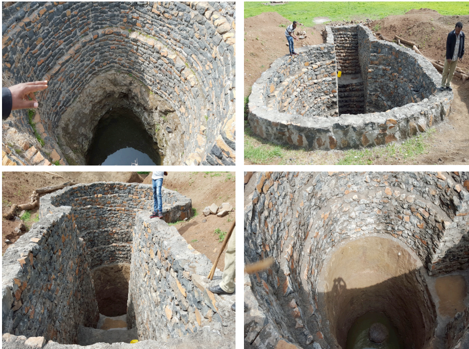
Figure 7 Stone masonry lining of HDWs and staged entrance ( Humera area, Ethiopia)
