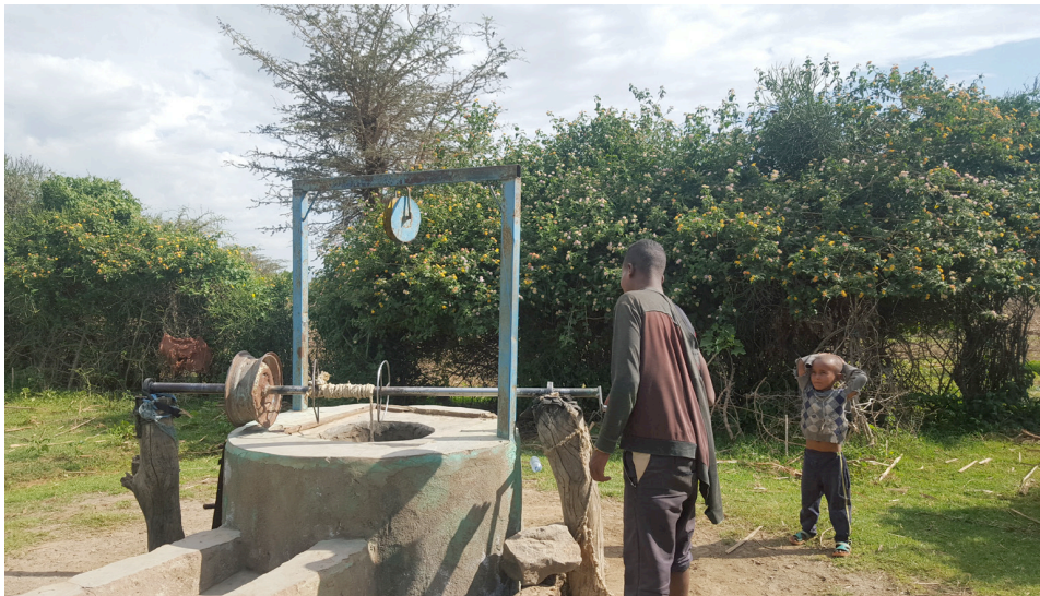
Figure 10 HDW equipped with manual pulley system changed to roller fitted with bearings attached with livestock cattle trough.
