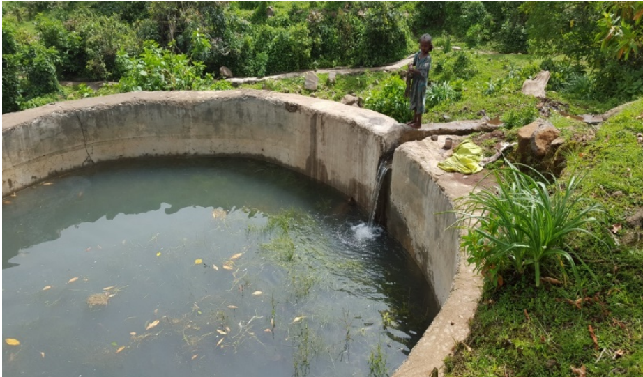
Figure 6-6 Night storage Reservoir (Embaguhalit-Tsegedie)
