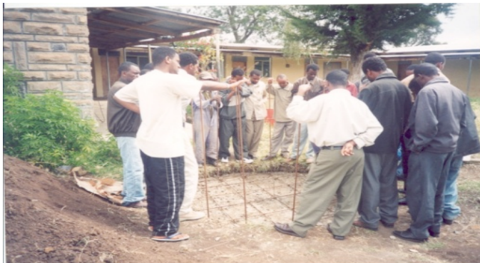
Figure 15: step 10-Fero cement rain water tank construction
