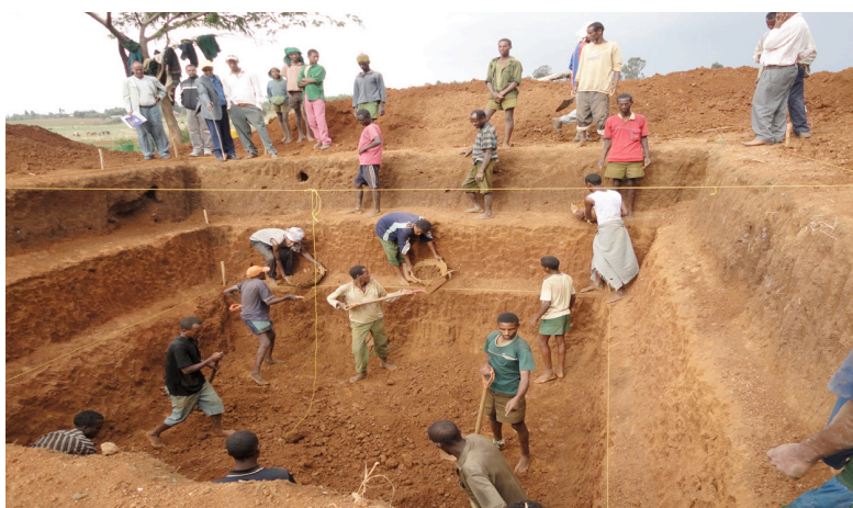
Figure 16: Stepwise construction on-going based on the layout made
