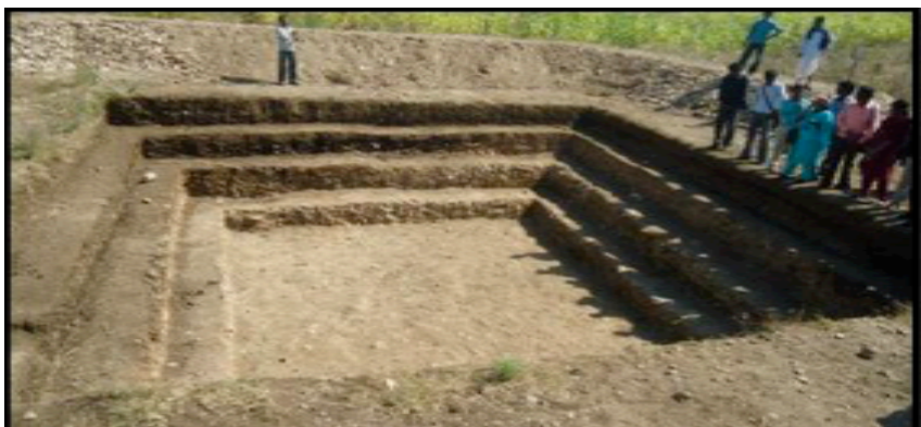
Figure 17: Stepwise digging, deepening and shaping the inner side of the pond surface
