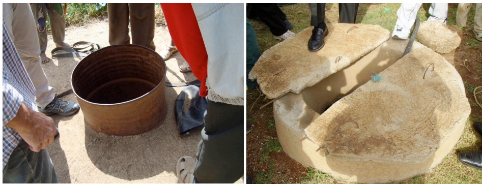
Figure 9 Head capping using metal barrel (left) and concrete (right)
