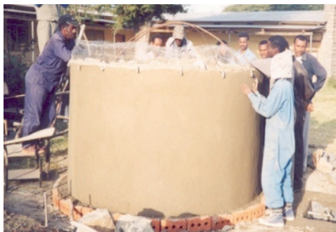
Figure 19: Step 19-Fero cement rain water tank construction
