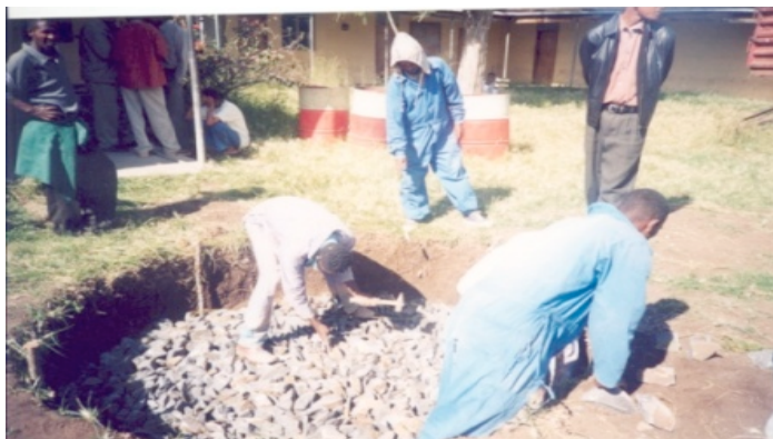
Figure 12: step 6-Fero cement rain water construction
