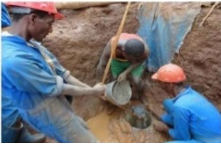
Figure 19: Gravel Pack filter
