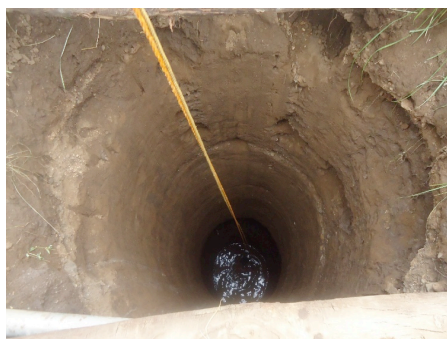
Figure 15 Excavated well before lining
