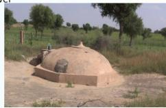
Photo- 2:- concreat covered subsurface water storage
