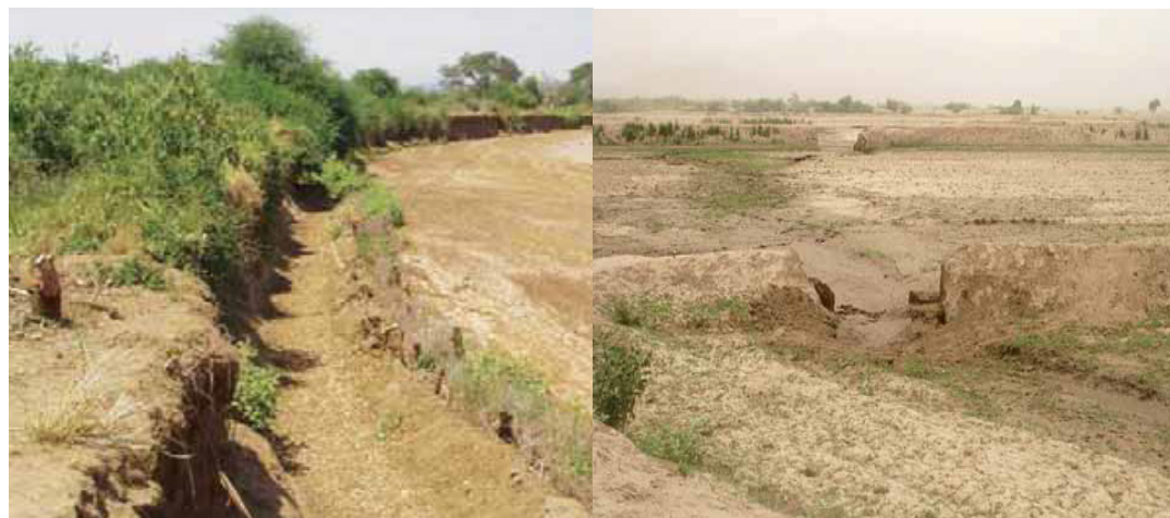
Figure 4.5: Traditional spate irrigation intake in Ethiopia (a) Field to field water distribution (Source FAO, 2010)
