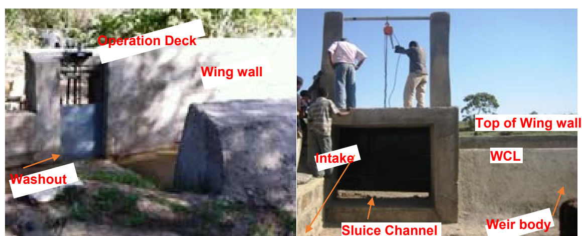
Figure 3-37: Washout gate operated by Spindle (L) and sluice gate by chain block (R)
