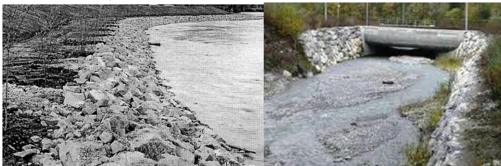
Figure 5-7: Rock riprap (L) and protection by gabion at u/s of river crossing (R)
