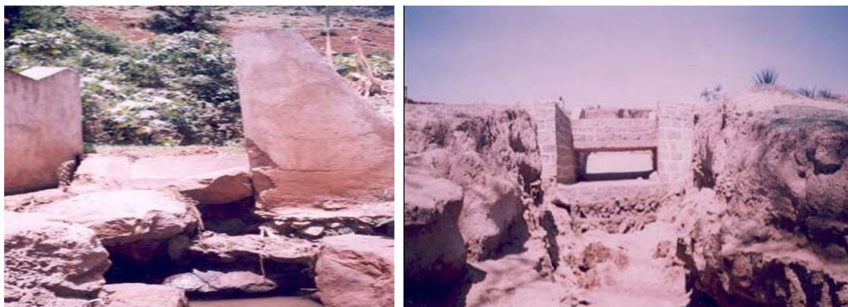
Figure 2-12: Collapsed weir as a result of piping (L) & scouring & absence of wings (R)
