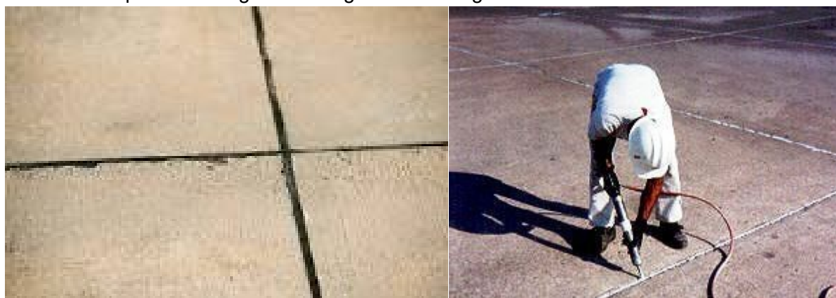
Figure 4-1: Sealant as seen in joints of concrete slabs
