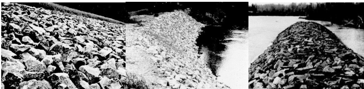
Figure 3-27: Dumped or hand-placed or plated riprap, HEC-11, 1997
