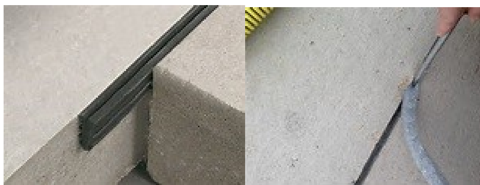
Figure 4-2: Joint fillers in concrete works
