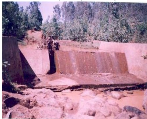
Figure 3-15: Insufficient Basin Length as Resulted in d/s Retrogression (SNNPR)
