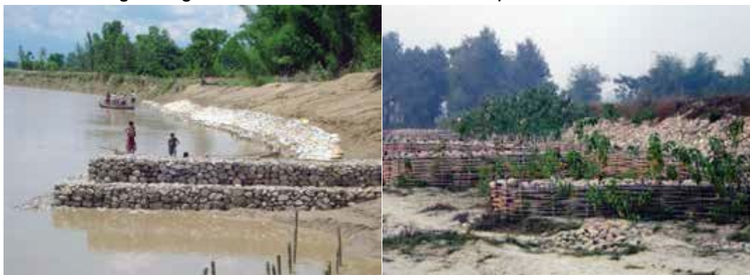
Figure 5-1: Arrangement of groynes along river bank, gabion (L) Bamboo (R)
