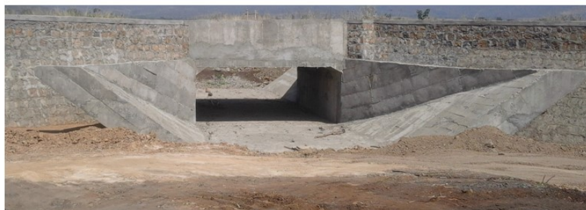
(a) Super passage under construction Viewed along the Irrigation Canal
