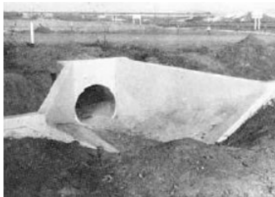
Figure 4-33: Photographic view of broken back concrete transition (Type-I) inlet & outlet
