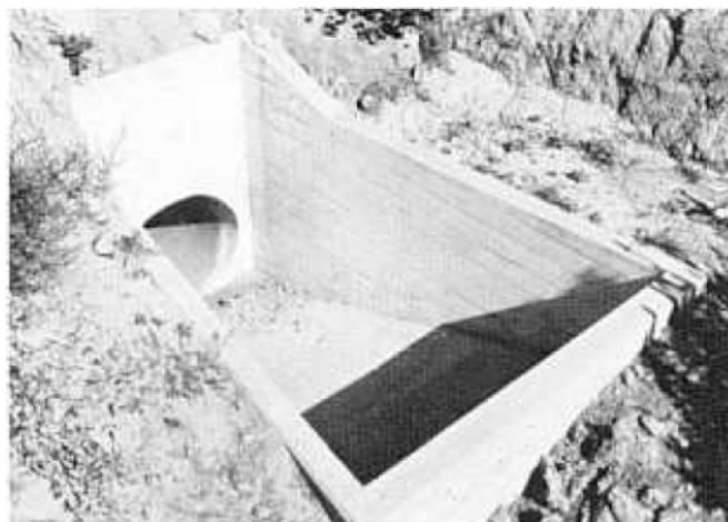
Figure 4-39: Photographic view of transition Type-IV inlet and outlet
