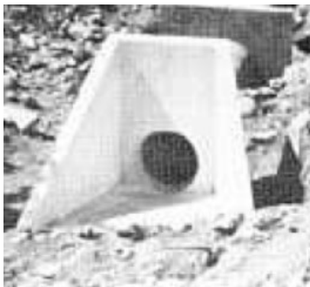
Figure 4-35: Photographic view of transition type-II inlet and outlet
