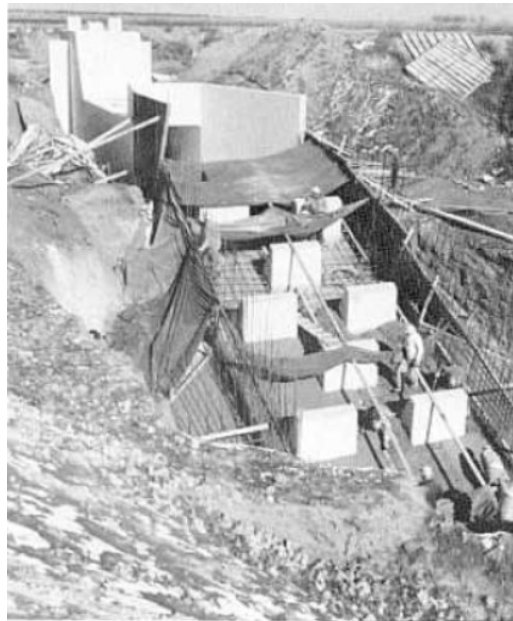
Figure 4-42: Baffled apron drop at concrete box culvert outlet
