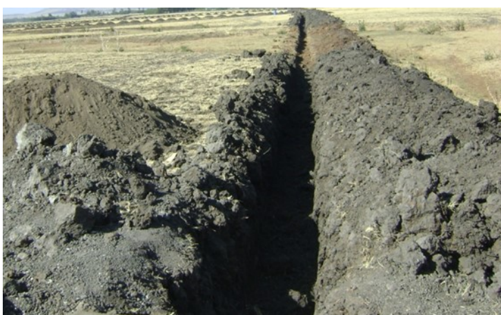
Figure 5-1: Trench for pipe laying
