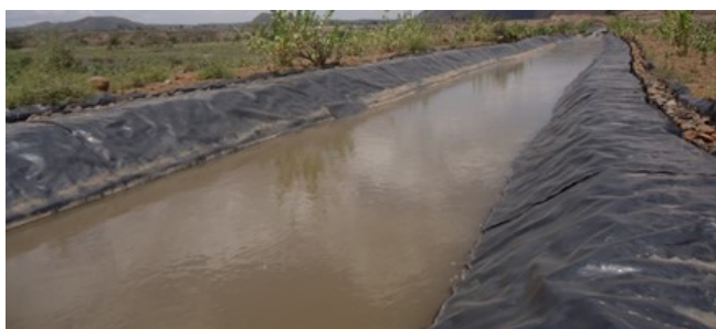
Figure 6-3: Main Canal Lined by Geo-membrane
