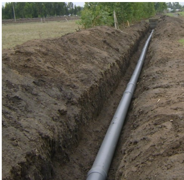
Figure 5-5: Pipe laying
