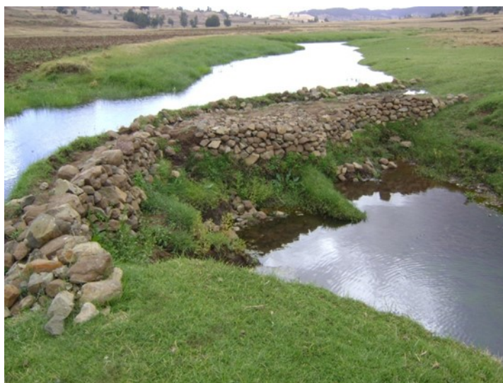
Figure 5-7: Cofferdam made of soil and stone
