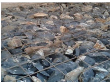
Figure 5-2: Hard core laying
