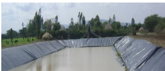
Figure 6-4: Night Storage Reservoir Lined by Geo-membrane
