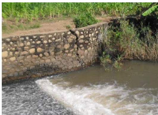
a) Wing wall that need repair
