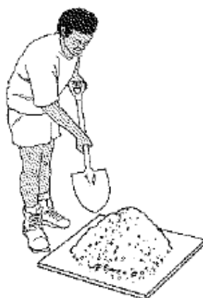
Figure 9-7: sand, cement and aggregate measured on mixing plate
