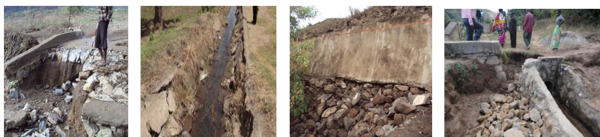
a) Washed by flood b) Collapse of stone wall c) Collapse of one side wall d) Wash out of division point
