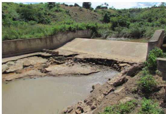
b) Headwork that need rehabilitation
