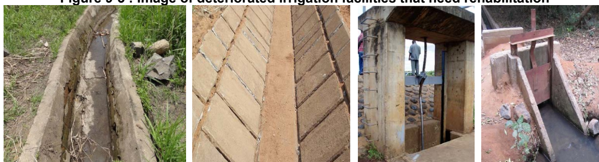
a) Abrasion wear of plaster b) Loss of joint mortar c) Deformed spindle d) deform of gate
