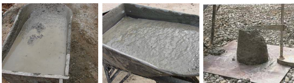
Figure 9-10: Images of hand mixed concrete
