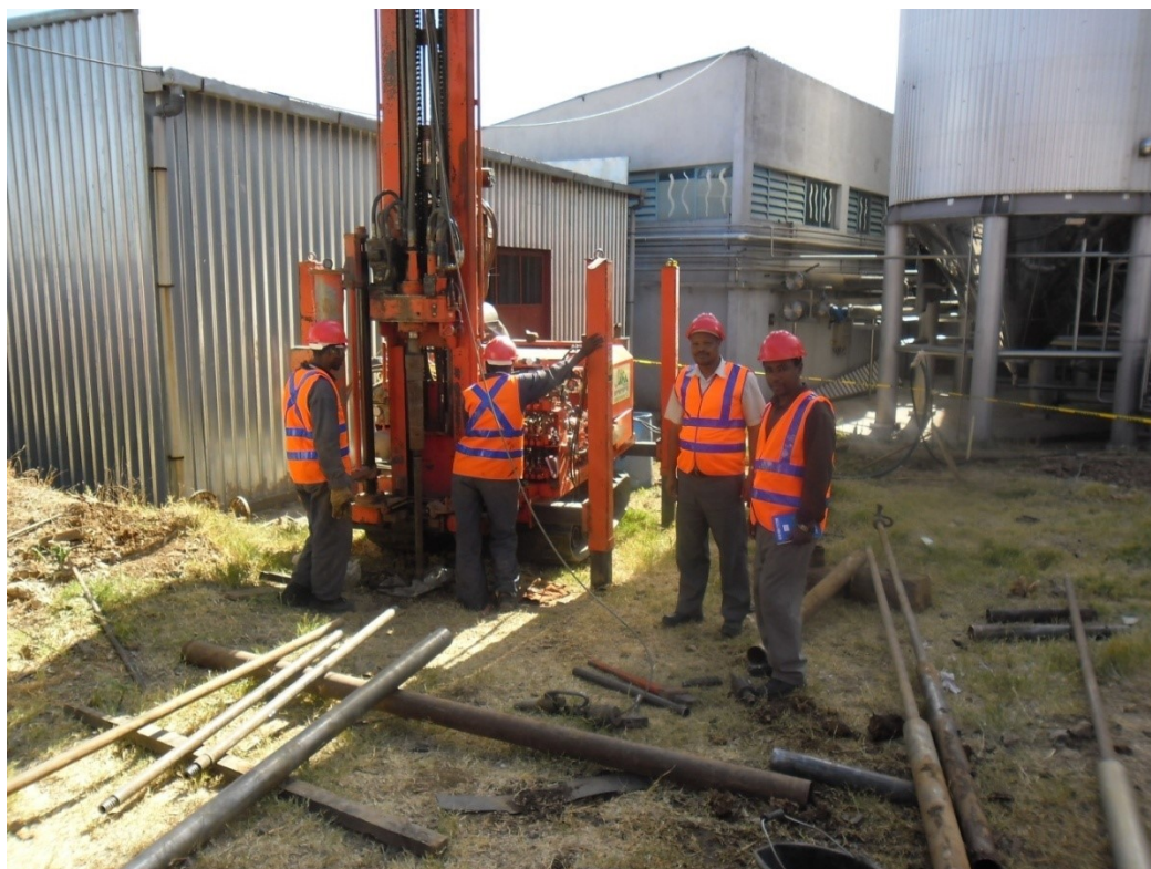
Figure 3-1: showing rotary core drilling at one of foundation Investigation site (drilling rig and accessories)
