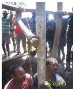
While installing 3" GIP casing
