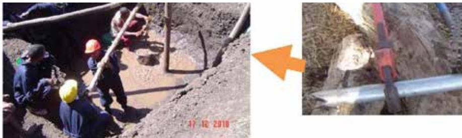
Figure 45: Use of Additional Tools for Hard Formation
