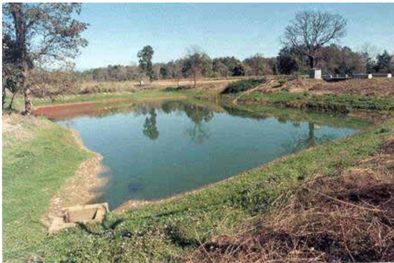
Figure 122: Percolation Tank (Spreading Basin)
