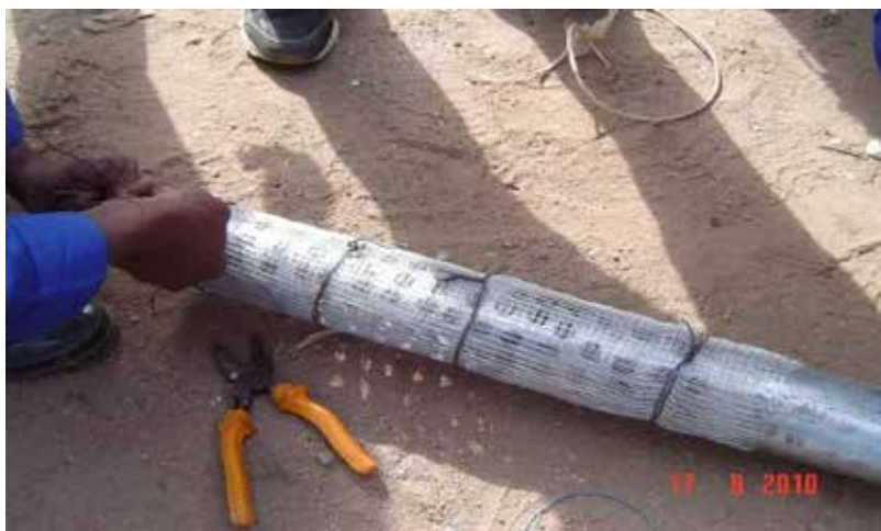
Figure 54: Perforated Screen with Screen Wire Mesh
