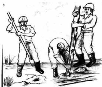
Figure 35: Erecting Wooden Poles
