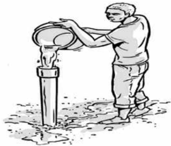
Figure 73: Cleaning Well and Flushing
