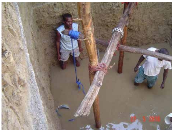
Figure 41: Tying Drilling Pipe and Sludge Lever with Nylon Rope or Chain (6 mm)
