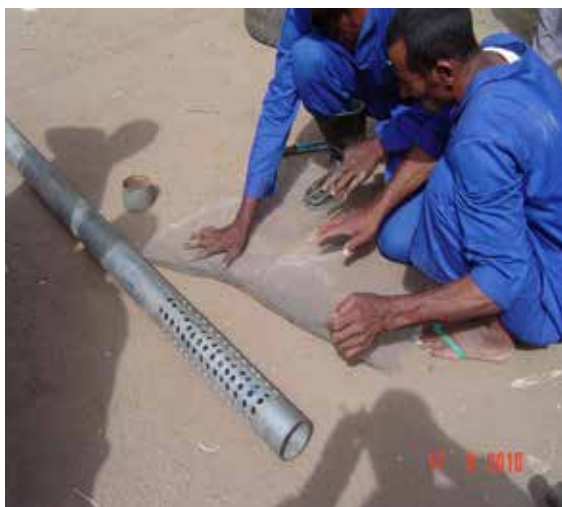
Figure 53: Type of Perforated Screen Casing
