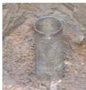
3" GIP casing prepared for diesel pump installation
