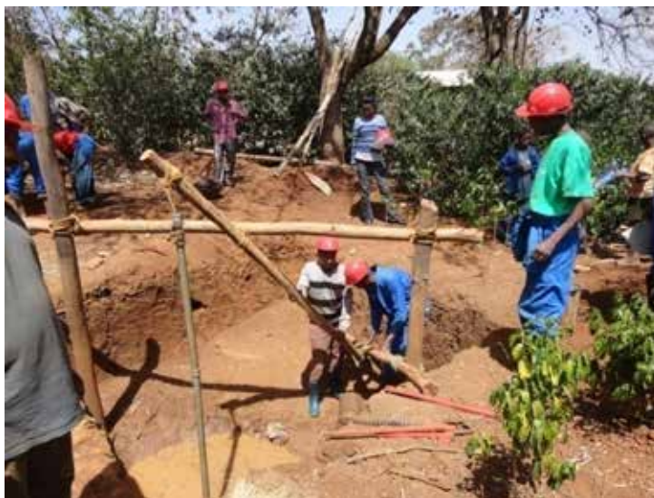
Figure 48: Hanging the Drilling Tools while at Rest
