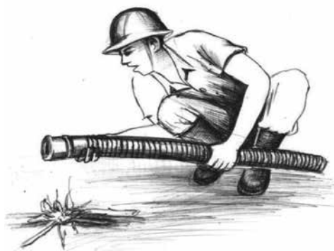
Figure 80: Process of Pump Installation (heating PVC for ease connection)
