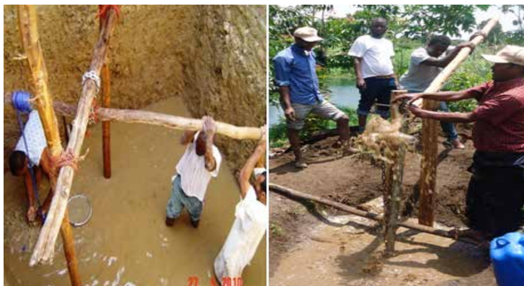
Figure 18: Simple Sludge Well Drilling Method
