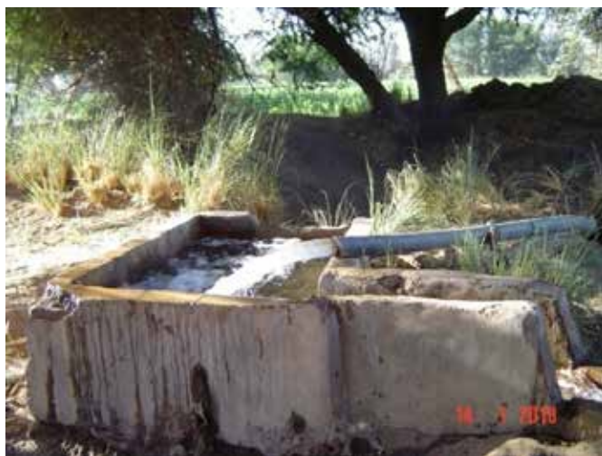
Figure 96: Delivery Pool with Masonry Structure
