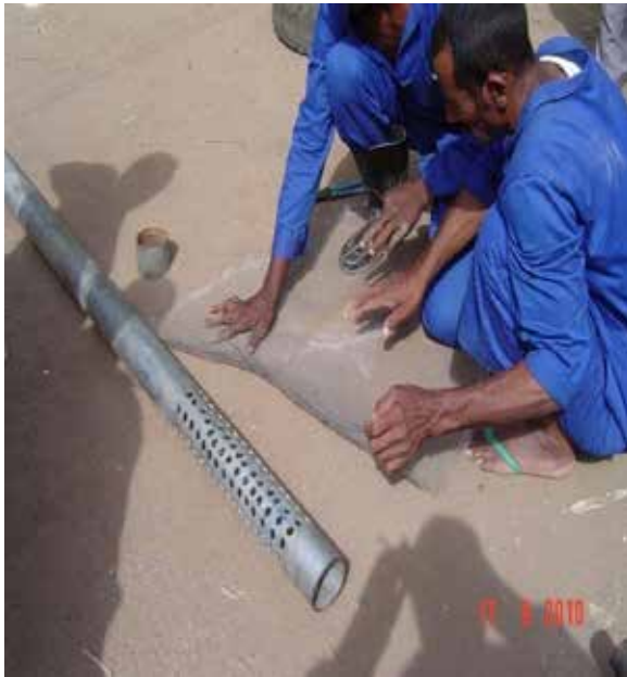
Figure 52: Blind and Screen Combined in one Casing
