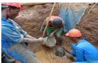
Figure 61: Pouring Gravel Pack
