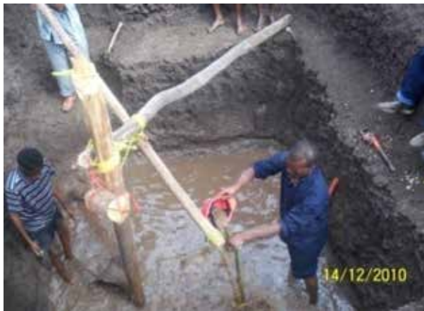
Figure 42: Priming the Drilling Pipe
